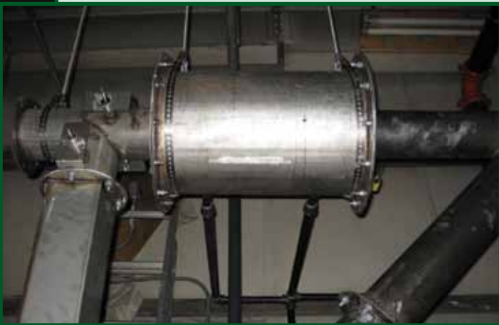
The air-to-water heat exchanger, which uses furnace exhaust to heat a 500-gallon water tank
